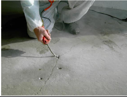
Setting injection packers
